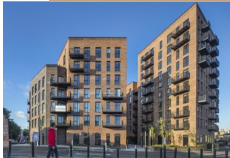
Figure 7: Dalston Works, London (Photo credit: Ramboll UK)
